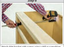
Attach slide bracket with screws using a drill or screwdriver.
